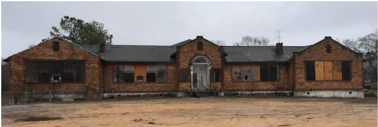
Thorsby Elementary School, Feb 2018, shortly before demolition.
